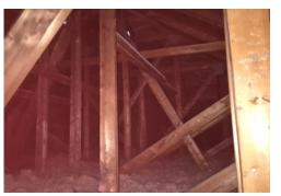
Comments: some minor staining on north underside of sheathing though does not appear to be mould
